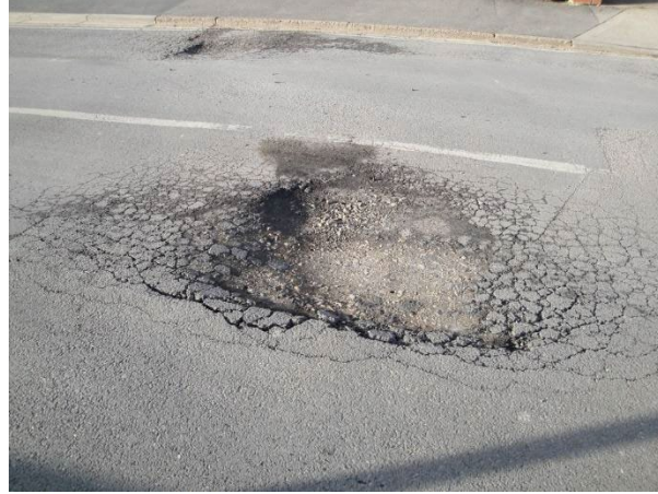
Figure 13.8: Thermal stress contributes to the formation of potholes. (credit: Editor5807, Wikimedia Commons)
