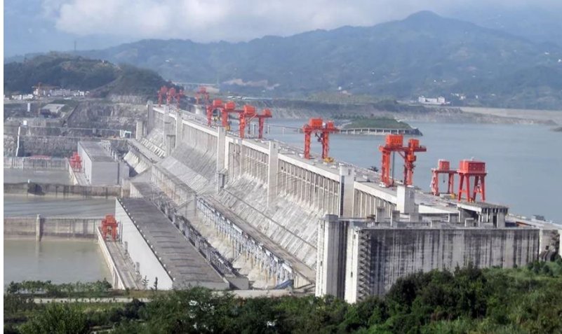
Figure 11.3: Three Gorges Dam in central China. When completed in 2008, this became the world's largest hydroelectric plant, generating power equivalent to that generated by 22 average-sized nuclear power plants. The concrete dam is 181 m high and 2.3 km across. The reservoir made by this dam is 660 km long. Over 1 million people were displaced by the creation of the reservoir. (credit: Le Grand Portage)
