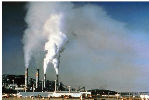
FIGURE 16.5 Air pollution billows from a power plant before the installation of emission control equipment for the removal of sulfur dioxide and particulate matter. Can you see why uncontrolled pollution is an example of the
