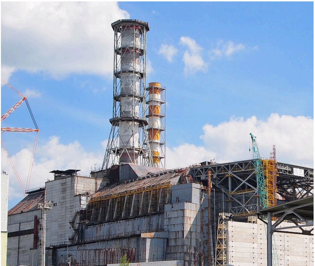
Figure 1. Today, Reactor #4 of the Chernobyl Nuclear Power Plant is encased in a sarcophagus to help contain radioactive material.
