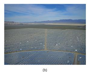
**Figure 9.10** (a) The Ivanpah solar thermal plant uses 170,000 mirrors to concentrate sunlight on water-filled towers. (b) It covers 4000 acres of public land near the Mojave Desert and the California-Nevada border. (credit a: modification of work by Craig Dietrich; credit b: modification of work by "USFWS Pacific Southwest Region"/Flickr)
