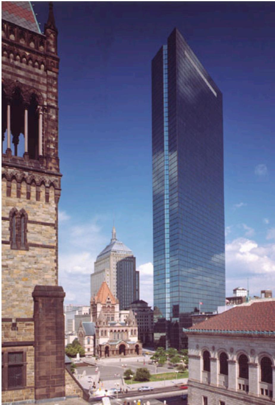
Figure 5.5.2 The John Hancock Tower
