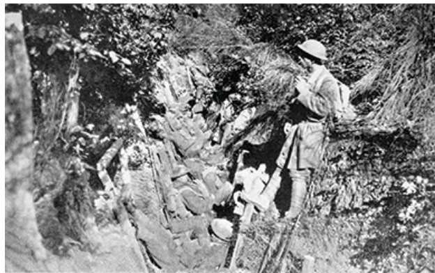
Figure 23.17 This photograph of U.S. soldiers in a trench hardly begins to capture the brutal conditions of trench warfare, where disease, rats, mud, and hunger plagued the men.
