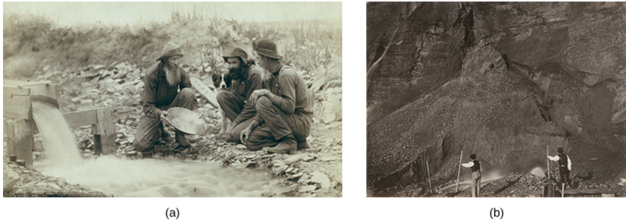
Figure 17.9 The first gold prospectors in the 1850s and 1860s worked with easily portable tools that allowed anyone to follow their dream and strike it rich (a). It didn't take long for the most accessible minerals to be stripped, making way for large mining operations, including hydraulic mining, where high-pressure water jets removed sediment and rocks (b).
