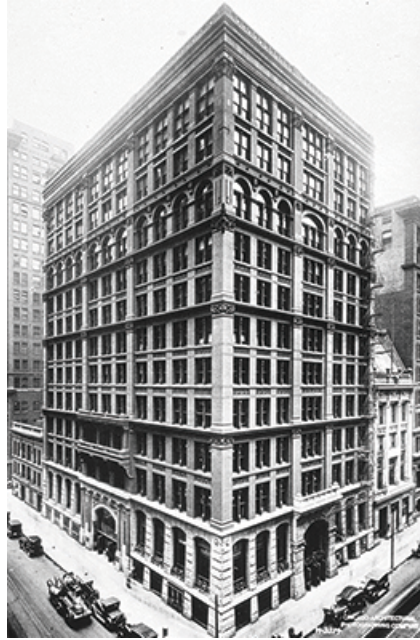
Figure 19.5 While the technology existed to engineer tall buildings, it was not until the invention of the electric elevator in 1889 that skyscrapers began to take over the urban landscape. Shown here is the Home Insurance Building in Chicago, considered the first modern skyscraper.
