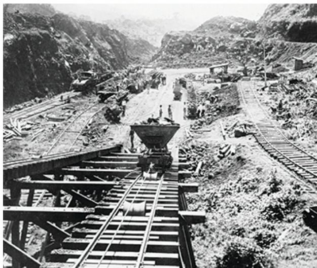
Figure 22.15 Recurring landslides made the excavation of the Culebra Cut one of the most technically challenging elements in the construction of the Panama Canal.
