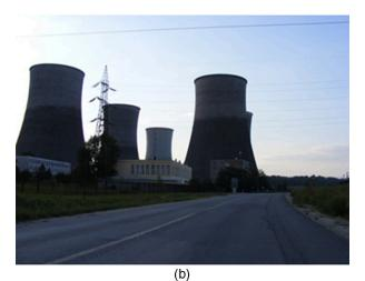
Figure 15.24 (a) A nuclear power station (credit: BlatantWorld.com) and (b) a coal-fired power station. Both have cooling towers in which water evaporates into the environment, representing  $Q_c$ . The nuclear reactor, which supplies  $Q_h$ , is housed inside the dome-shaped containment buildings. (credit: Robert & Mihaela Vicol, publicphoto.org)
