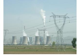
Figure 7.24 Tremendous amounts of electric power are generated by coal-fired power plants such as this one in China, but an even larger amount of power goes into heat transfer to the surroundings. The large cooling towers here are needed to transfer heat as rapidly as it is produced. The transfer of heat is not unique to coal plants but is an unavoidable consequence of generating electric power from any fuel—nuclear, coal, oil, natural gas, or the like. (credit: Kleinolive, Wikimedia Commons)
