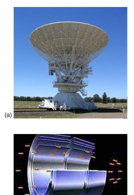
Figure 26.26 (a) The Australia Telescope Compact Array at Narrabri (500 km NW of Sydney). (credit: Ian Bailey) (b) The focusing of x rays on the Chandra Observatory, a satellite orbiting earth. X rays ricochet off 4 pairs of mirrors forming a barrelled pathway leading to the focus point. (credit: NASA)
