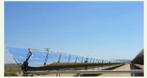
Figure 25.44 Parabolic trough collectors are used to generate electricity in southern California. (credit: kjkolb, Wikimedia Commons)
