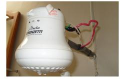
Figure 20.41 On-demand electric hot water heater. Heat is supplied to water only when needed. (credit: aviddavid, Flickr)
