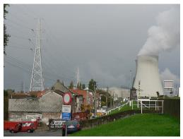
Figure 32.22 The people living near this nuclear power plant have no measurable exposure to radiation that is traceable to the plant. About 16% of the world's electrical power is generated by controlled nuclear fission in such plants. The cooling towers are the most prominent features but are not unique to nuclear power. The reactor is in the small domed building to the left of the towers. (credit: Kalmthouts)
