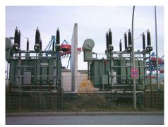
Figure 20.19 Power is distributed over large distances at high voltage to reduce power loss in the transmission lines. The voltages generated at the power plant are stepped up by passive devices called transformers (see Transformers) to 330,000 volts (or more in some places worldwide). At the point of use, the transformers reduce the voltage transmitted for safe residential and commercial use. (Credit: GeorgHH, Wikimedia Commons)
