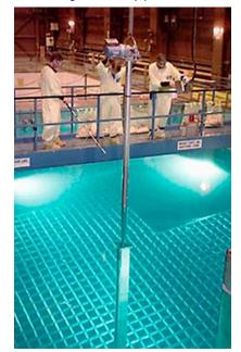
Figure 14.32 Radioactive spent-fuel pool at a nuclear power plant. Spent fuel stays hot for a long time. (credit: U.S. Department of Energy)
